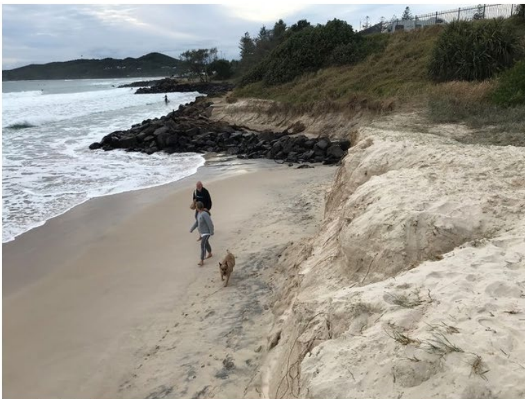
Recent 'end effect' erosion at Main Beach seawall.
