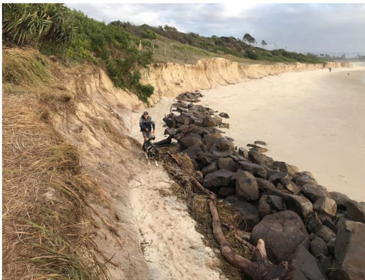
Storm cut erosion west of Main Beach seawall
