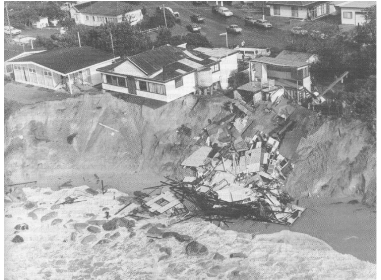
Figure 1 Erosion at Terrigal Beach 20th June 1978. House collapses on the high tide at 8.00 a.m. The House to the left collapsed on the subsequent high tide at 10.10 p.m. (photo courtesy of News Limited).
